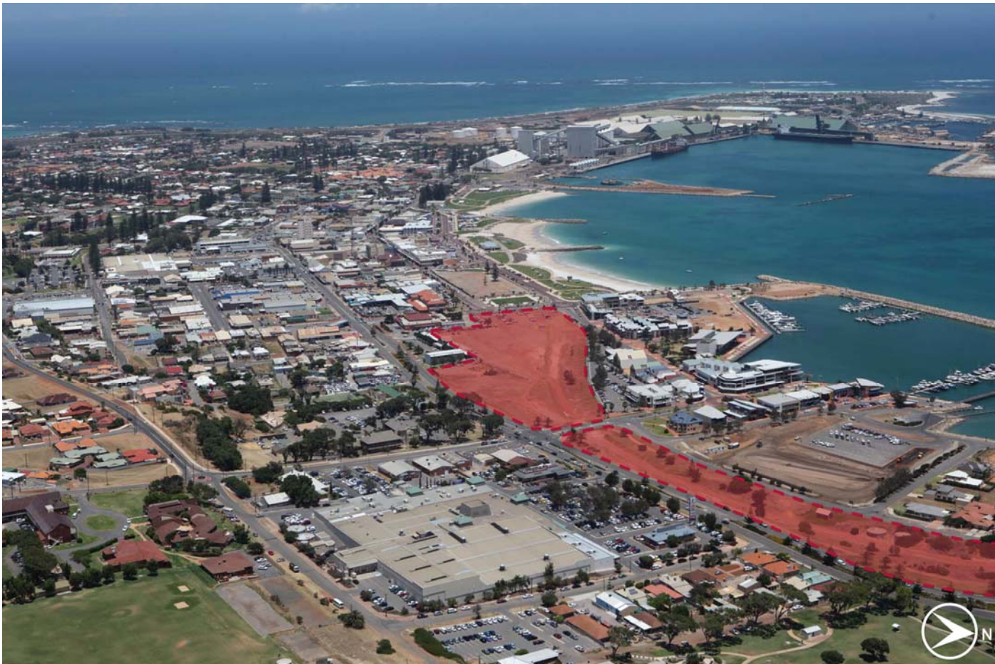
Geraldton Coast looking south -west across Batavia Coast Marina Stage 2
