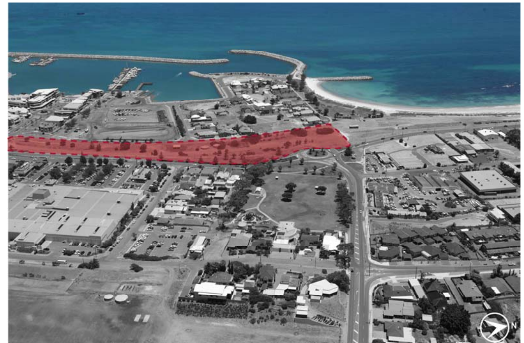
Geraldton Coast looking north-west across the northern extent of Batavia Coast Marina Stage 2
